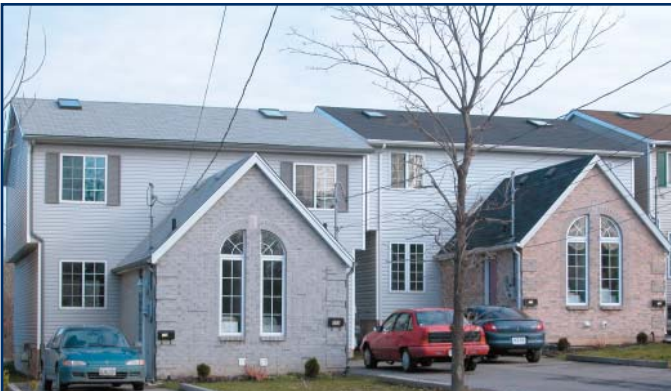
In a Brock University study conducted by Dr. Tony Shaw, the house on the left (built with SIPs) was 33% more energy efficient than the house on the right (built with traditional lumber framing)
