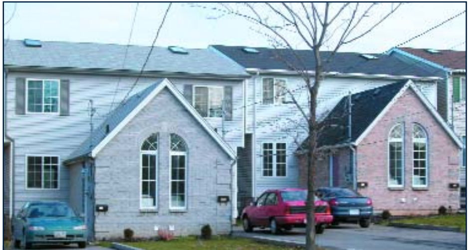
Dr. Tony Shaw of Brock University compared the thermal efficiency of two units in these nearly identical semi-detached homes. The house on the left was built with SIPs, while the other was framed with studs and batt insulation.
